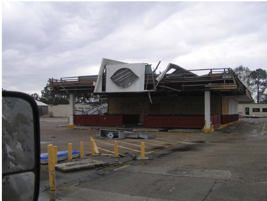
Damage to a Dairy Queen in Winnie TX. Photograph was taken on the afternoon of September 15, 2008 by Tanya Brown.
