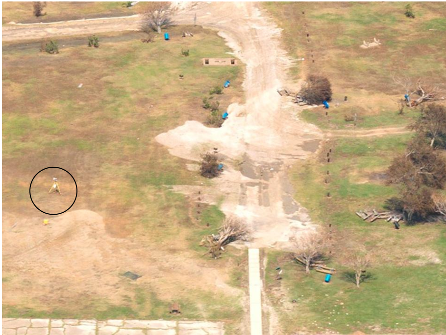
Aerial photograph of Probe 0110A (circled) on the grounds of Ft. Travis on the western end of the Bolivar Peninsula. Even though the area was inundated with approximately 2 ft of storm surge (which overtopped the fort's seawall of 17 ft.) the probe continued to operate collecting data for seven and a half days. Photograph courtesy of ABS Consulting.
