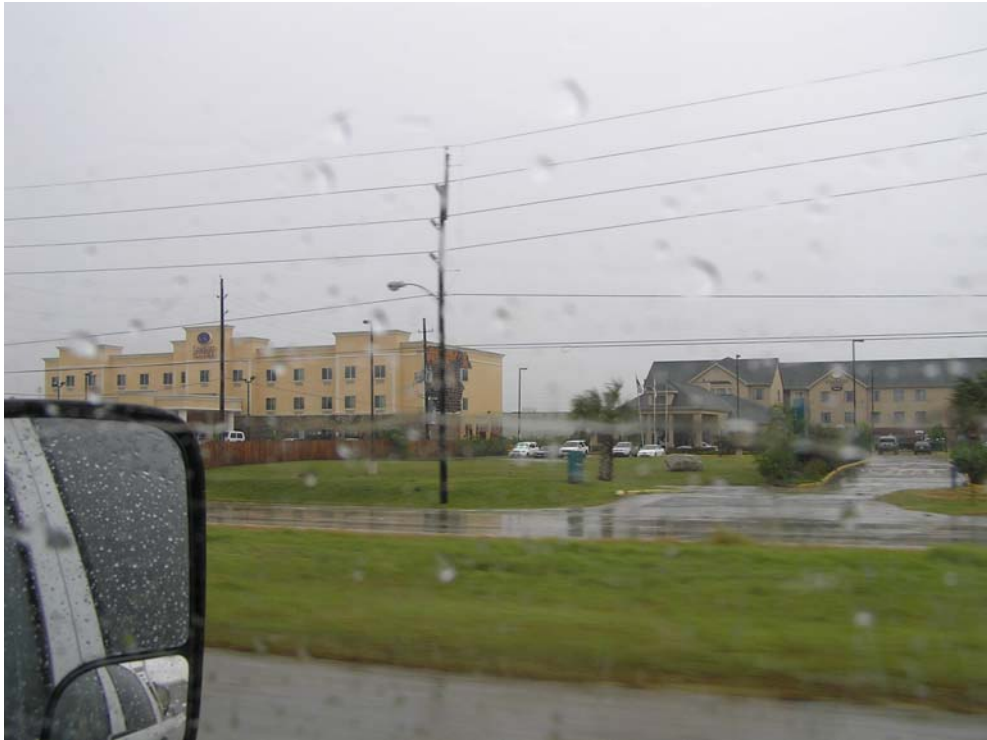
Hotel siding damage east of Houston. Photograph taken 9:00 am CDT September 14, 2008. Photograph by Tanya Brown.
